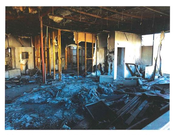
Photograph 3: Signs of fire damage inside the building - ceiling and floor (01/08/19).
